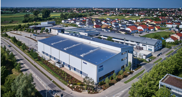
The Sonplas GmbH site in Straubing
